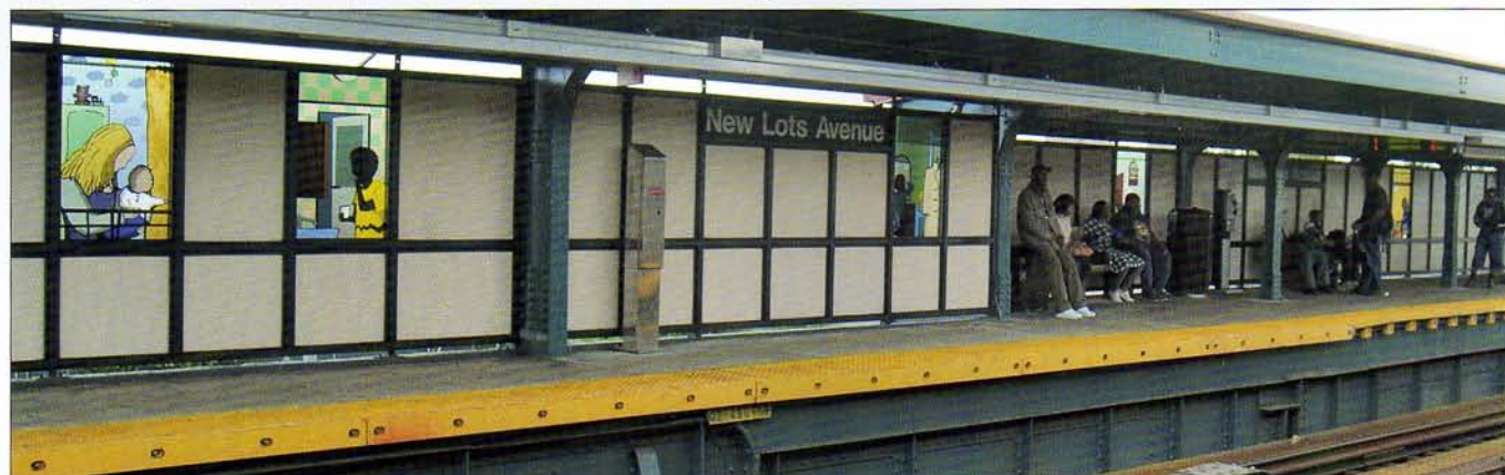
Eugenie Tung, Windows , 2007. A platform view of the installation showing the Manhattan Bound platform, where the „Day“ panels are installed.
